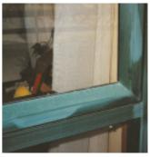
Examples of solvent misuse on aluminium joinery, showing  $\,$  deterioration of powder coating after 3 years.
